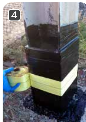
4 Kevlar® and epoxy resin wrap
