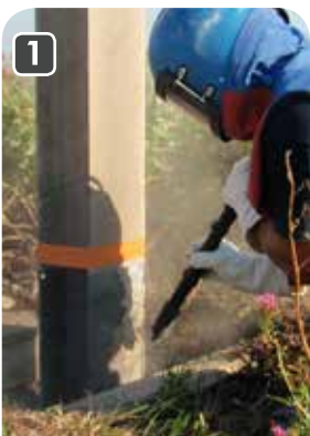
1 Surface preparation Sa2½
